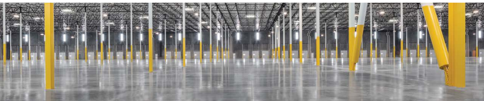
IMCO Real Estate portfolio: 1.2 million square feet of modern, best-in-class logistics space fully leased to a large, global logistics and supply chain company with over 1,000 employees in 35+ countries worldwide, located in Glendale, Arizona. Image by WPT Capital Advisors
