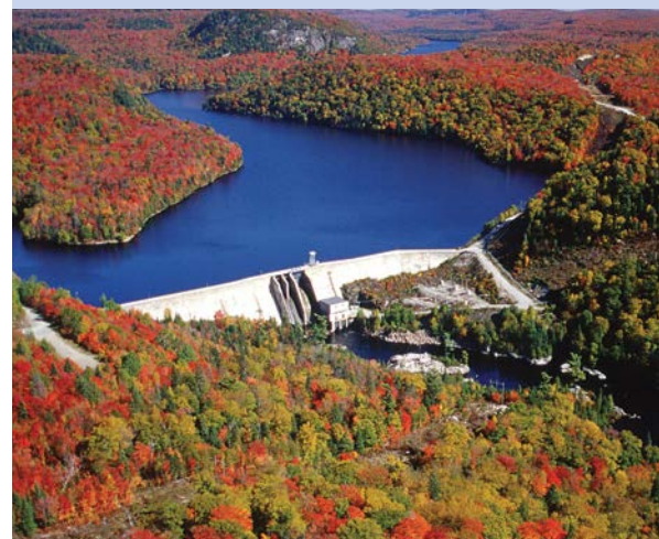
Aerial view of a hydroelectric dam in Gartshore, Ontario. Image by Brookfield
