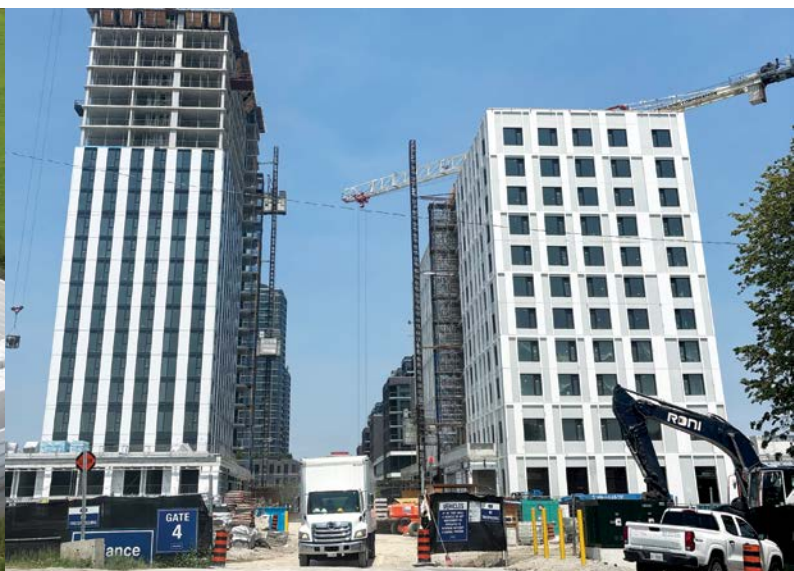
West Square under construction in Toronto, Ontario. Image by KingSett Capital
